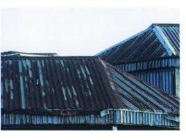
The useful life of chrysotile cement roofing is about twice that of iron roofing, depending on the type of corrosion protection used.
